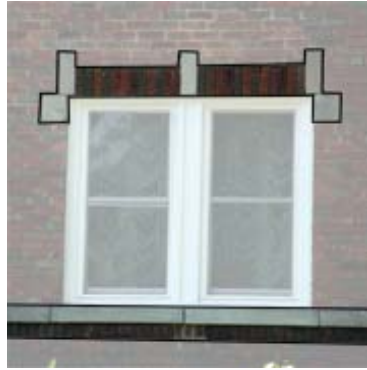
(stone windowsills & stone detailing above windows)
