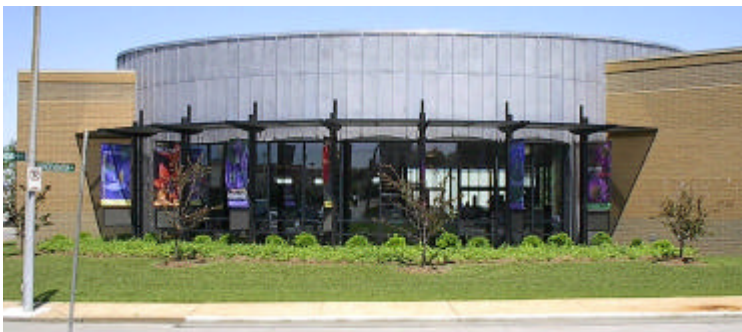
Kingshighway Library at 2260 South Vandeventer
